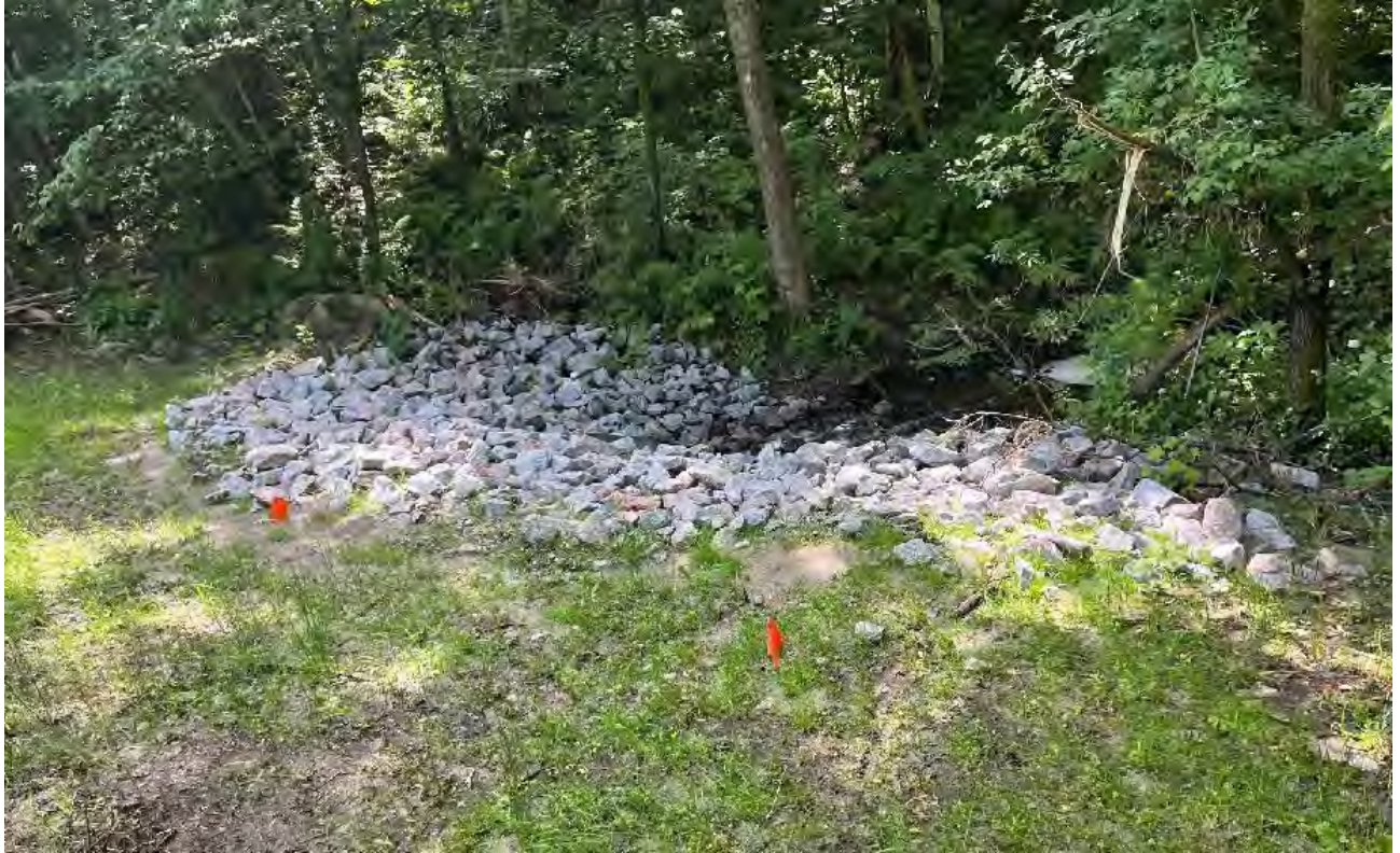
Birchdale Township culvert/outlet stabilization project
